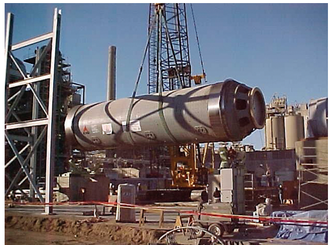
220 ton cement kiln refurbishment done with Twin-Path®
